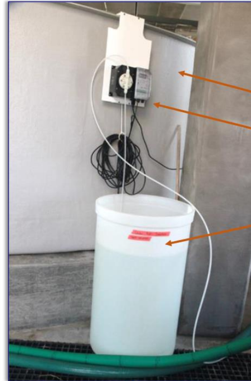
Delivering a buffering solution into a water storage tank using a pH controller and pump
